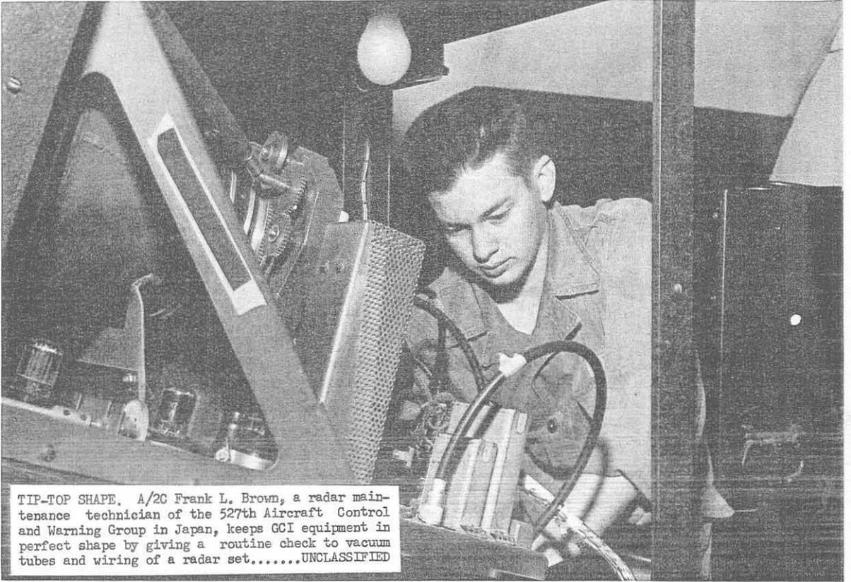
TIP-TOP SHAPE. A/2C Frank L. Brown, a radar maintenance technician of the 527th Aircraft Control and Warning Group in Japan, keeps GCI equipment in perfect shape by giving a routine check to vacuum tubes and wiring of a radar set.....UNCLASSIFIED
